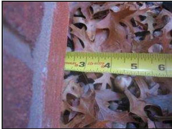
3.0 Picture 1 - Top center of rear basement wall.
